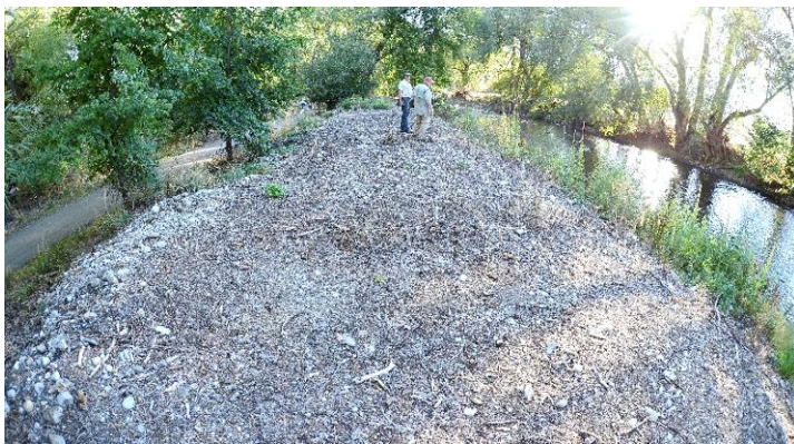
Figure A2: Photo of dredge pile levee along the bank of the Logan River in the Golf Course. Logan River is located to the right in the picture.
